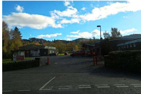
Telephone Exchange, Keswick Telereal Trillium
