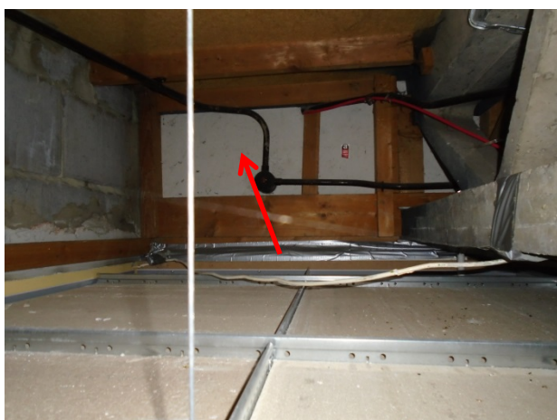
Photograph 19: G.28 Kitchen – Asbestos insulating board (AIB) fire break between G.13 Corridor and G.29 Café.
