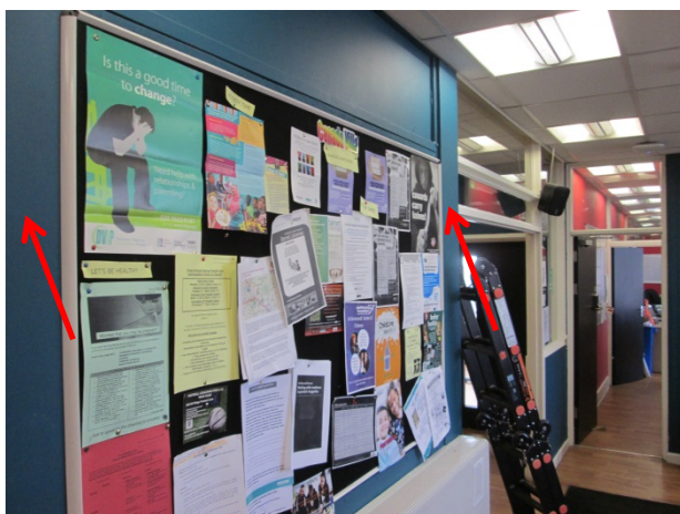
Photograph 1: G.01 Entrance Lobby – Asbestos Insulating Board (AIB) panels identified to wall, over-clad with MDF.
