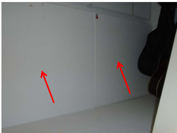
Photograph 13: G.22 Small Teaching Room – Asbestos insulating board (AIB) ceiling panels.
