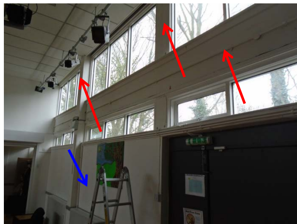
Photograph 14: G.24 Main Hall – Asbestos insulating board (AIB) wall panels below window positions to external wall. Asbestos insulating board (AIB) inset panels to walls.
