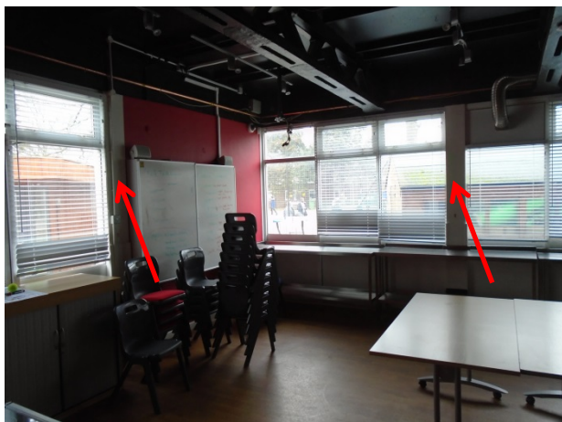
Photograph 21: G.29 Café - Asbestos insulating board cladding to metal columns, AIB over-clad with MDF.
