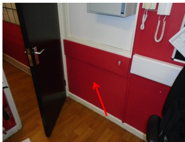
Photograph 4: G.04 Main Office – Asbestos insulating board (AIB) infill panel below window into G.14 Gym.
