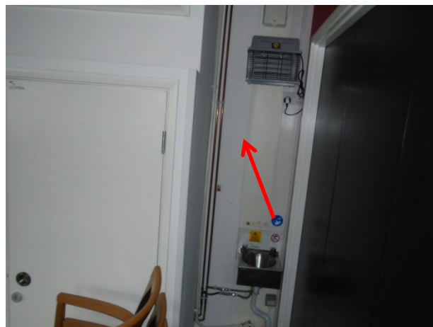
Photograph 22: G.29 Café – Asbestos insulating wall panelling to G.14 Gym wall present behind modern cooker units.
