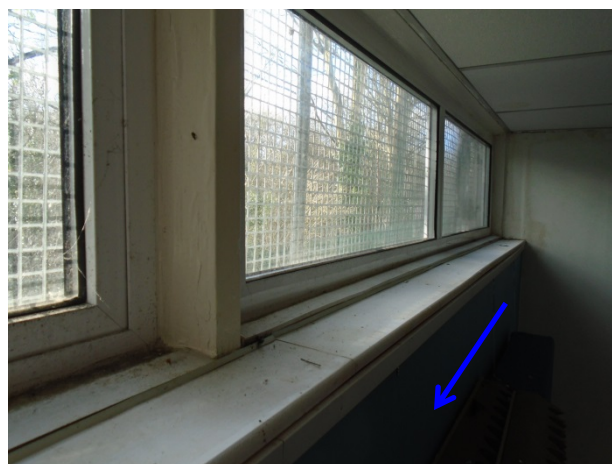
Photograph 12: G.19 Radio Booth – Asbestos insulating board (AIB) infill panels are suspected to be present to the external facing wall behind plasterboard.
