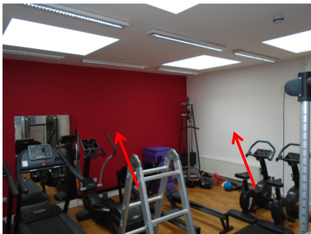
Photograph 9: G.14 Gym – Asbestos insulating board (AIB) panelling to low level window positions behind plasterboard wall lining.
