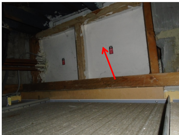
Photograph 18: G.28 Kitchen – Asbestos insulating board (AIB) door header panel within ceiling void.
