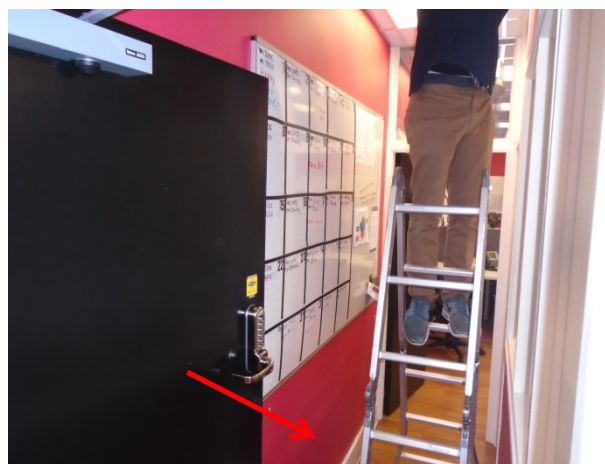
Photograph 2: G.02 Office Corridor -- Asbestos Insulating Board (AIB) infill panels previously identified below windows to G.14 Gym. Now over-clad.
