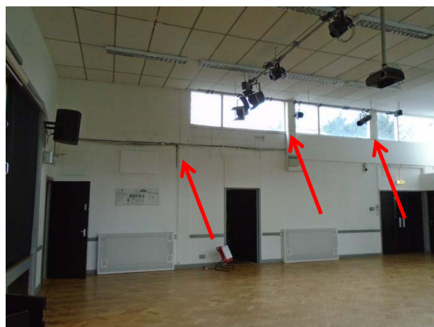
Photograph 16: G.24 Main Hall – Asbestos insulating board (AIB) inset panels to wall.
