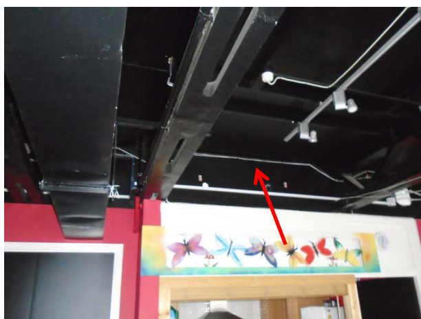
Photograph 20: G.29 Café - Asbestos insulating board firebreak to G.28 Kitchen ceiling void.
