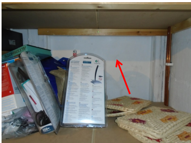
Photograph 17: G.27 'D of E' Store – Asbestos insulating board (AIB) door header panel above sealed doorway and timber infill.
