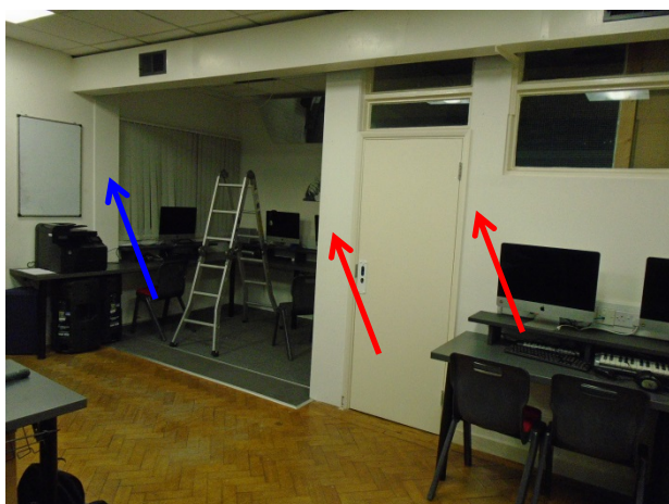
Photograph 11: G.18 Rithmik Music Studio – Asbestos Insulating Board (AIB) panels identified to wall, over-clad with MDF.
