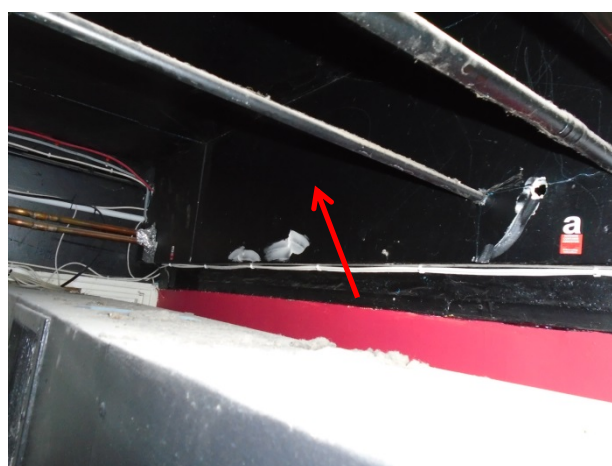
Photograph 8: G.13 Corridor – Asbestos insulating board (AIB) firebreak to high level wall between G.13 Main Corridor and G.28 Kitchen.
