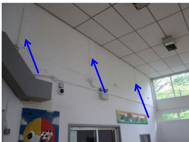
Photograph 15: G.24 Main Hall – Asbestos insulating board (AIB) inset panels to wall previously identified, now covered over by a mezzanine level extension; no evidence of removal works supplied at time of inspection, presumed to remain behind modern extension.
